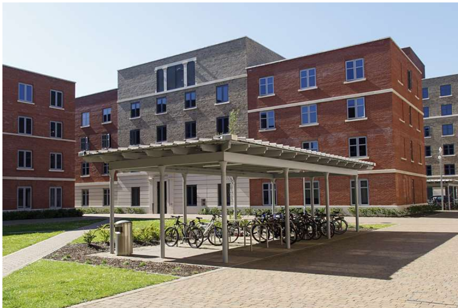
Figure 25 Sheltered Bike Storage
